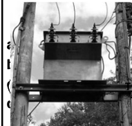
Three-phase, pole mounted "step down" Transformer
